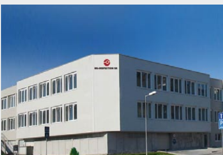
ME Inspection, Bratislava
